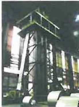
Cold rolling mill – ENTRY TOWER FOR ACCUMULATION
