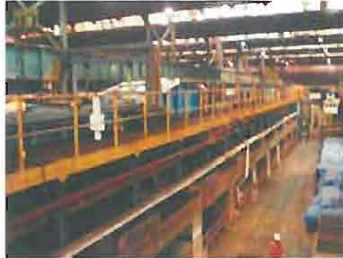
Cold rolling mill – CHEMICAL SECTION OF PICKLING LINE 1
