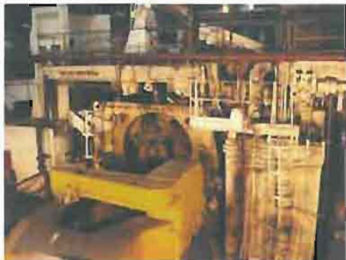
Hot rolling mill – COILER
